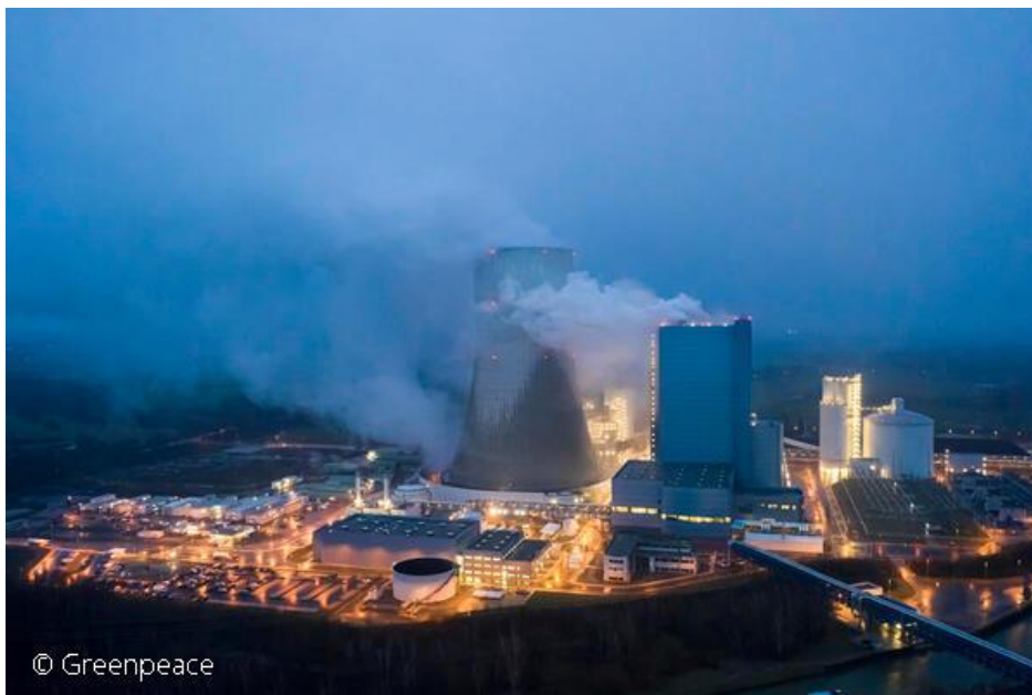
PHOTO: DATTELN 4 POWER STATION IN GERMANY
