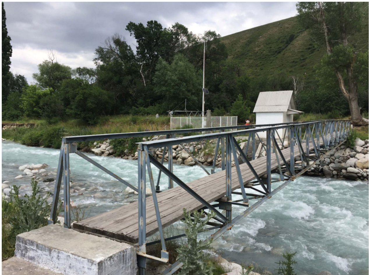
Bridge to enable profiling at the Baityk Station on the Alaarcha River, Kyrgyz Republic. Source: D. Kull, 2017.
