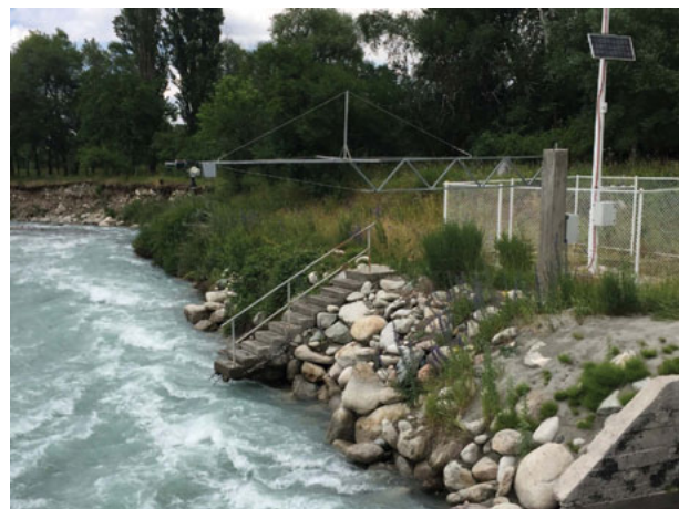
River monitoring equipment at the Baityk Station on the Alaarcha River, Kyrgyz Republic. Source: D. Kull, 2017.
