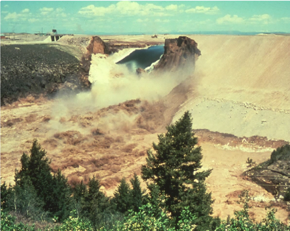
Significant Turbulence and Sediment load during the Teton Dam Failure
