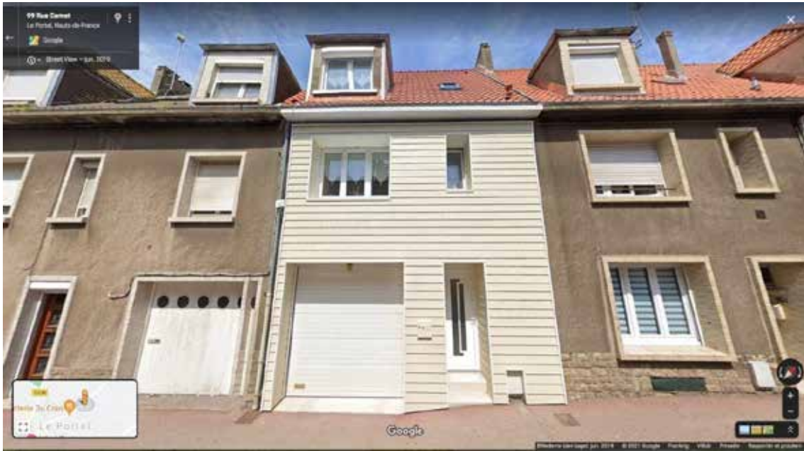
Figure 2. External wall insulation in PVC, Le Portel, © Google Street maps.
