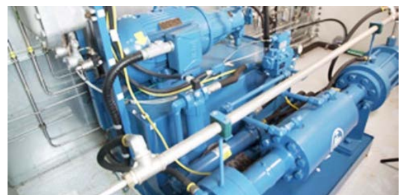
Figure 4. HydroPac compressor.
