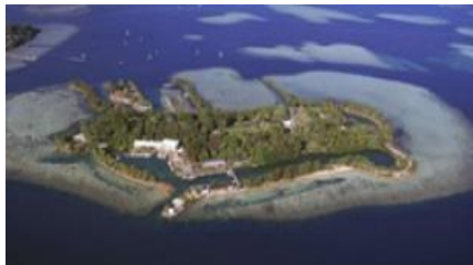
Figure 1. DC microgrid project site, Coconut Island.
