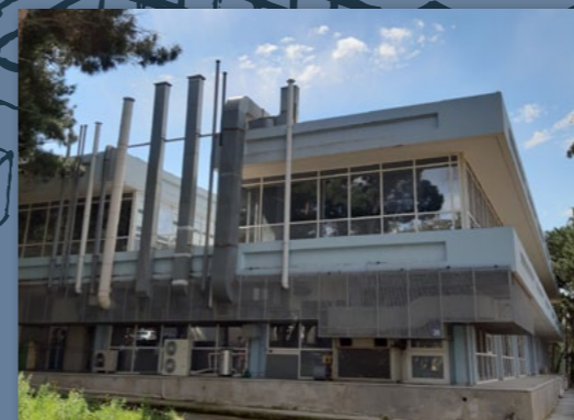
Existing IIT Building
