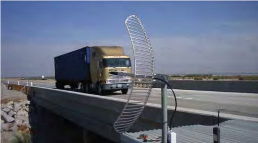
Kings Stormwater Channel Bridge on Route 86 in Riverside County is constructed of non-traditional and composite materials. Photo courtesy of http://hpwren.ucsd.edu .
