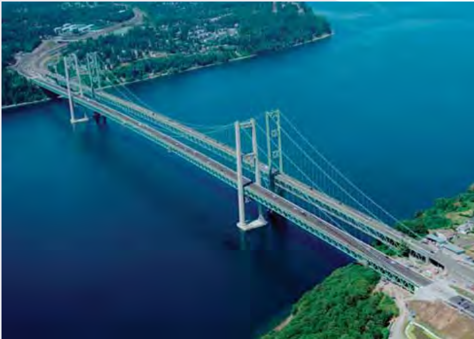
Completed Tacoma Narrows Bridge. Photo courtesy of Washington Department of Transportation.
