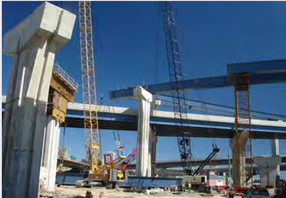
Marquette Interchange construction. Photo courtesy of Wisconsin Department of Transportation.
