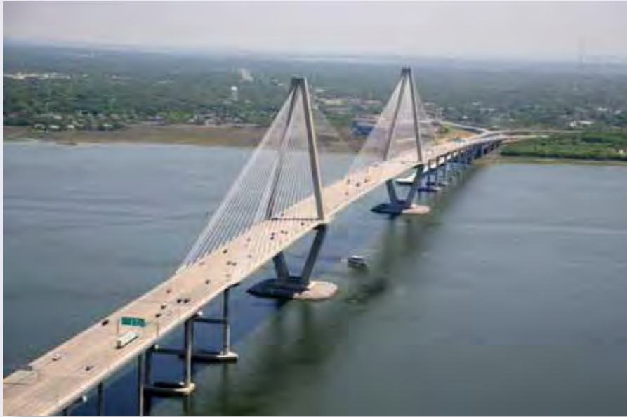
Cooper River Bridge. Photo courtesy of Rob Thompson, South Carolina Department of Transportation.
