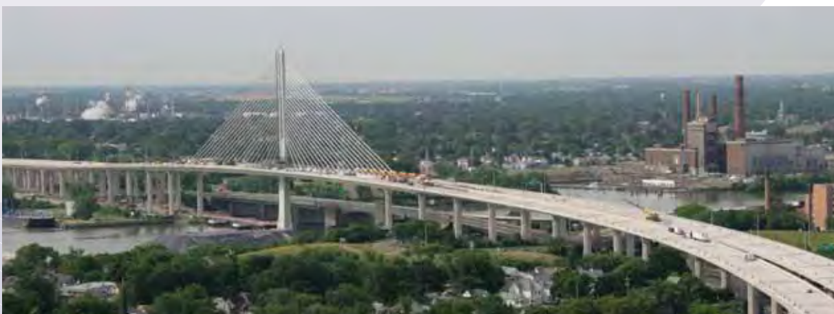
Veterans' Glass City Skyway in Toledo, Ohio. Photo courtesy of Ohio Department of Transportation
