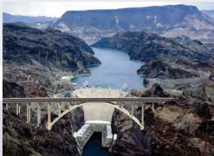
Rendering of the Mike O'Callaghan-Pat Tillman Memorial Bridge that will be built between Nevada and Arizona near the Hoover Dam. Photo courtesy of Nevada Department of Transportation
