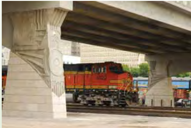
Demonbreun Street Bridge.
