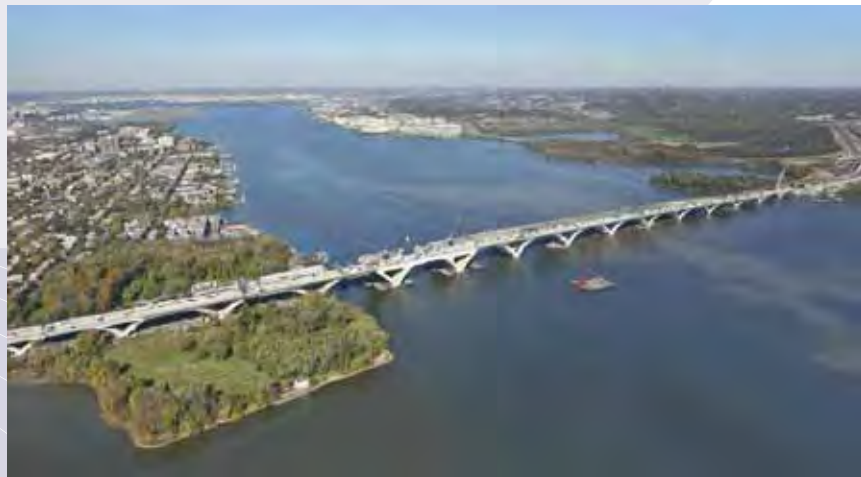
Woodrow Wilson Bridge Photo courtesy of Virginia Department of Transportation
