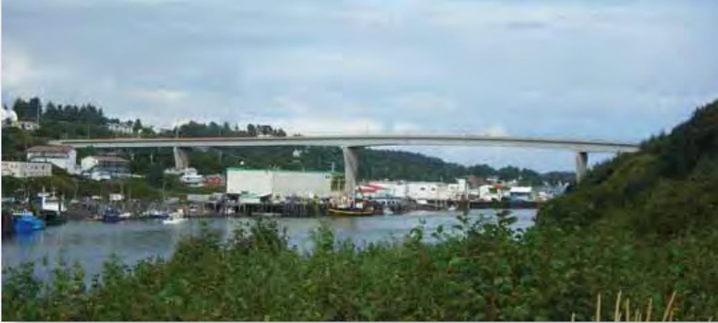
Kodiak Harbor Channel Bridge seismic retrofit. Photo courtesy of Alaska Department of Transportation and Public Facilities.
