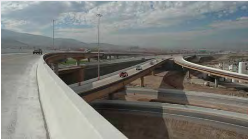
Nevada Spaghetti Bowl in Henderson Photo courtesy of Nevada Department of Transportation
