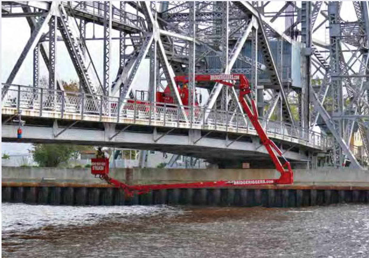
Snooper truck inspection. Photo courtesy of Duluth Shipping News.
