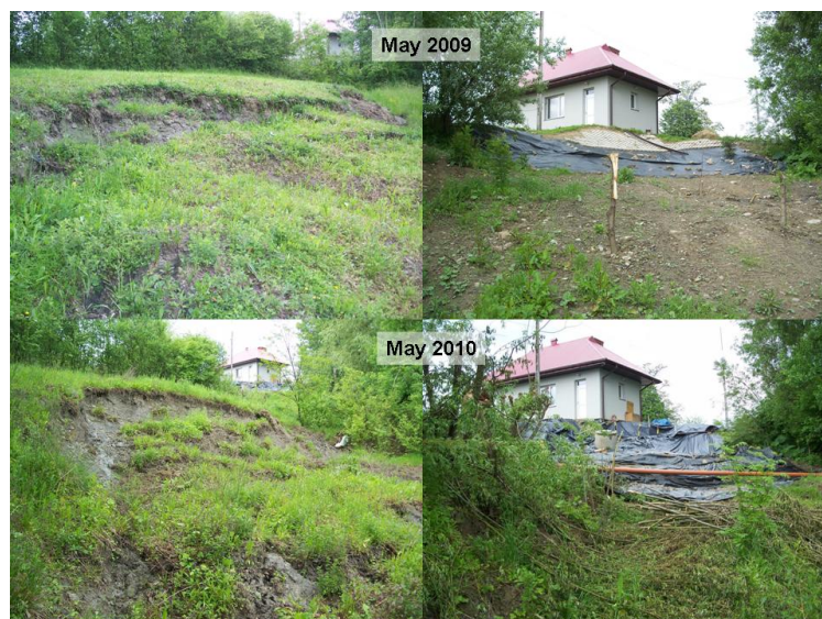
Fig. 6 Zbyszycze landslide in the direct neighborhood of the petrol station (Fig. 8).
