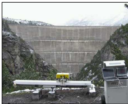
Fig. 6 – IBIS-L positioned in front of the downstream face of the Cancano dam (Alta Valtellina, Italy)
