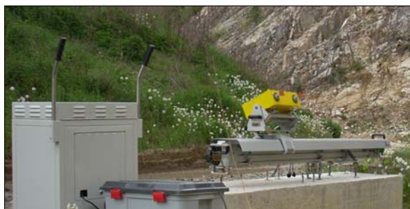
Fig. 1. IBIS-L system installed on a concrete foundation
