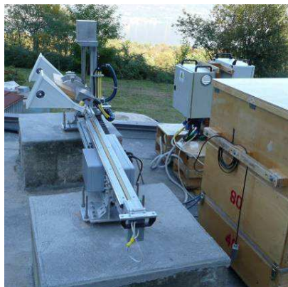
Figure 3. The GB-SAR instrument attached to mechanical frames fixed to two concrete bases realized on the building
