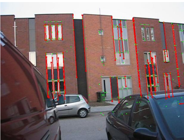
Figure 3. Matched 2D edges with reliable points, Reliable points (green), edges with end points (red) frame 0 (upper), frame 133 (lower)
