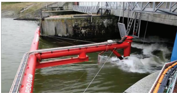
Figure 11 Example of testing in a Sluice gate (TTC, 2017)
