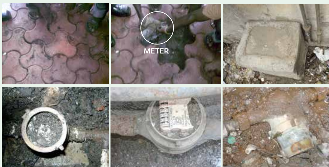
Figure 2. Examples of meter reading issues (clockwise from top left): Meter buried under footpath, enclosed in cement, broken meter, readings not accessible (Gomes, 2012; Itron India, 2009)
