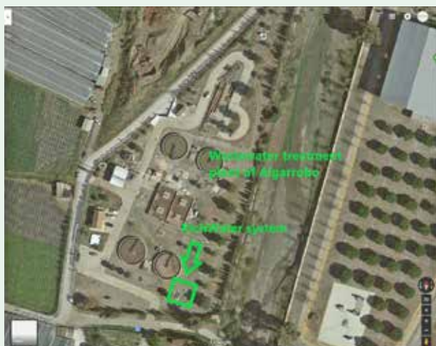
Figure 3. Algarrobo WWTP and RichWater MBR location
