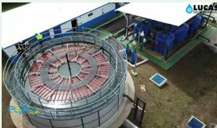
Figure 5. Breña Mora PWTP - Radial flow settlers with SDM (source: LE and ESPH)
