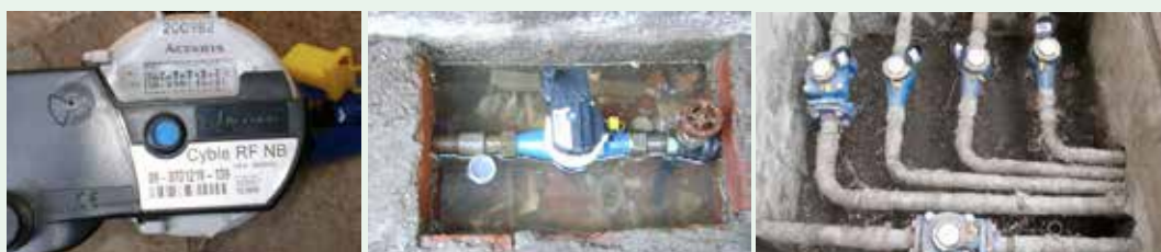
Figure 3. Installed AMR meters in Mumbai (Gomes, 2012)
