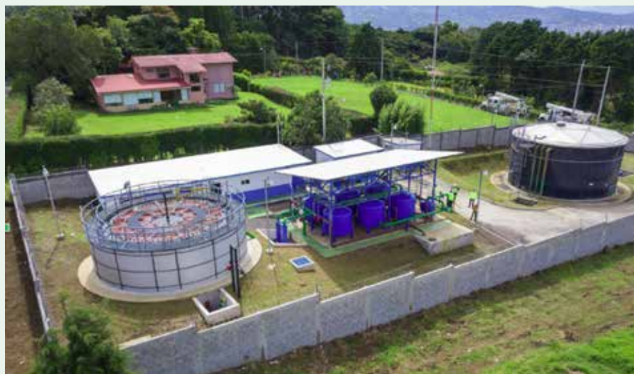
Figure 6. Full view of Breña Mora PWTP - Radial flow settlers with SDM (source: LE)
