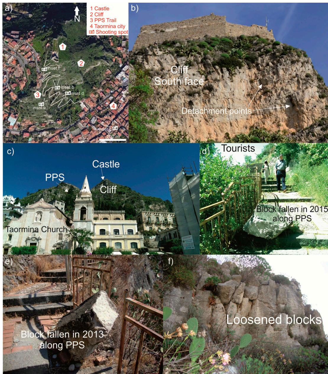
Figure 3. (a) Location of the main elements on a satellite image (PPS: panoramic pedestrian stairway); (b) a view of the Saracen Castle and the south face of the cliff; (c) panoramic view of the cliff from the main square of Taormina; (d) block fallen along PPS in 2015; (e) block fallen along PPS in 2013; (f) unstable, loosened blocks occurring along the cliff.
