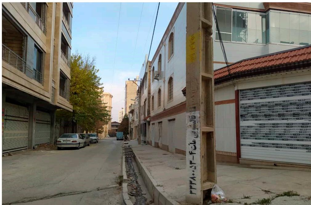
**Figure 2.** The lack of two-way drainage systems in most of the streets in the study area that can result in the inefficient collection of the rainfalls.
