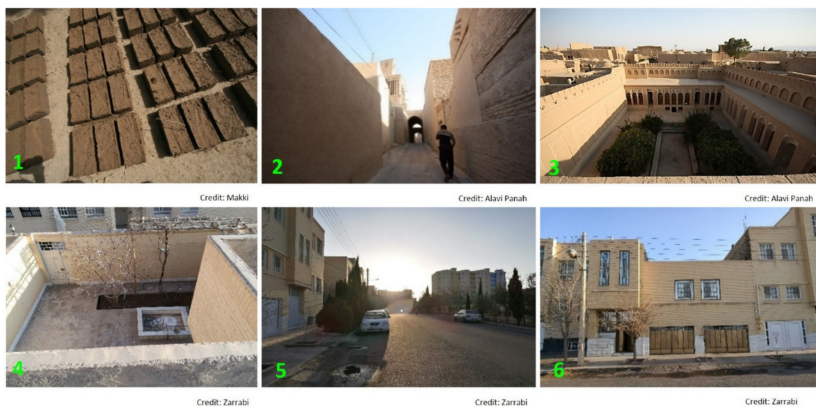
Figure 2. The physical morphology of the buildings in the historical district and the new district. Pictures 1–3 show the historical district, and pictures 4–6 show the new district of the city of Yazd. Picture 1 was taken by Mohsen Maki, pictures 2 and 3 were taken by Alavi Panah and pictures 4–6 were taken by Amirmasoud Zarrabi.
