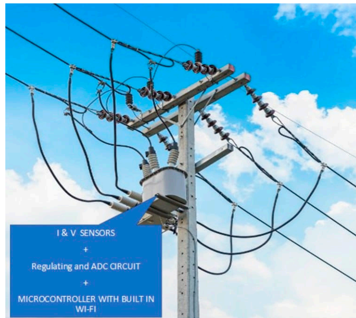
Figure 7. Transmission line monitoring subsystem.
