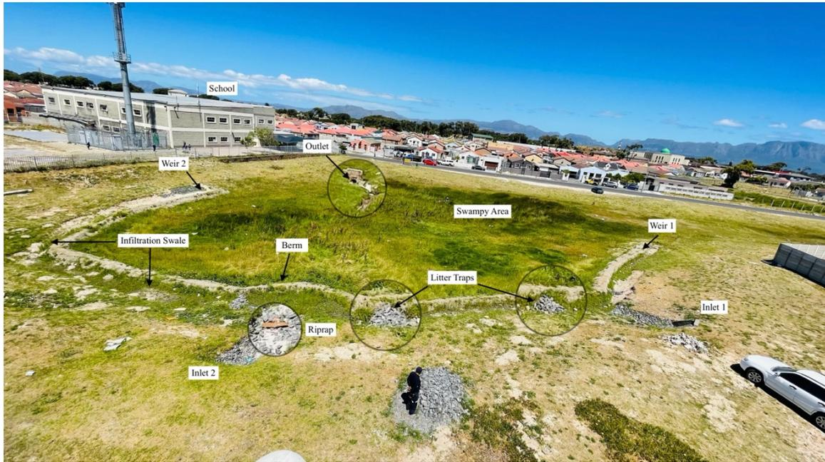
Figure 3. Retrofitted detention pond [11].
