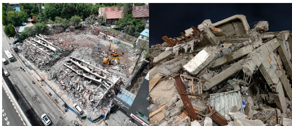
Figure 15. The muck pile of mechanical edifice.
