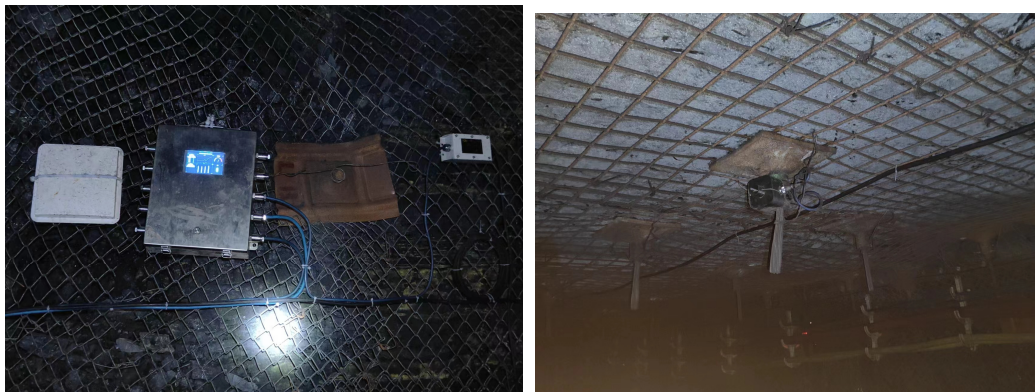
Figure 5. On-site installation of concentrators and sensors.
