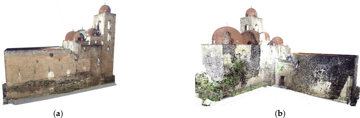
Figure 11. The final point cloud of St. John the Evangelist of the Hermits: (a) the east side, (b) the west side.
