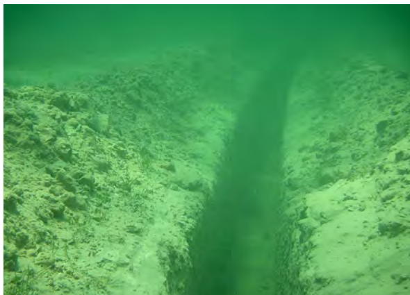
Figure 1 Cable trench on shallow sandy sea bottom
