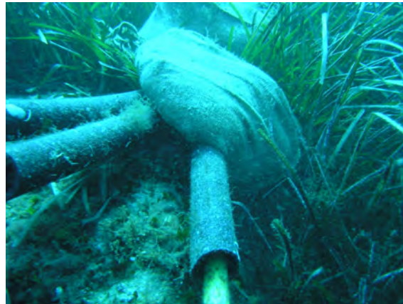
Figure 2 Optical cable coastal protection with a layer of sand-cement bags
