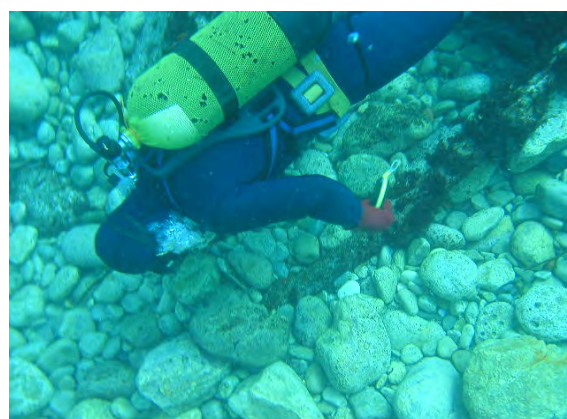
Figure 3 Optical cable maintenance on the seabed
