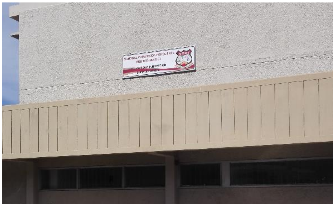
Figure 2: Technology and Innovation Support Centre within Lingadzi House
