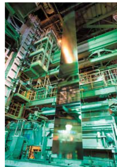
溶融亜鉛めっき設備 Continuous Galvanizing Line
