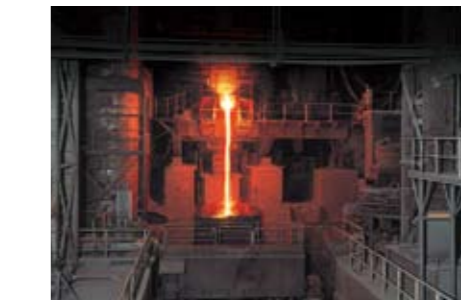
電気炉 (和歌山) Electric arc furnace (Wakayama Works)
