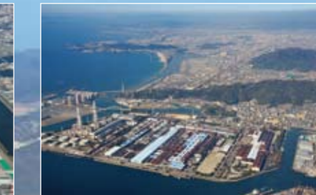
和歌山地区(海南) 全景 Overall view of [Kainan Area]
