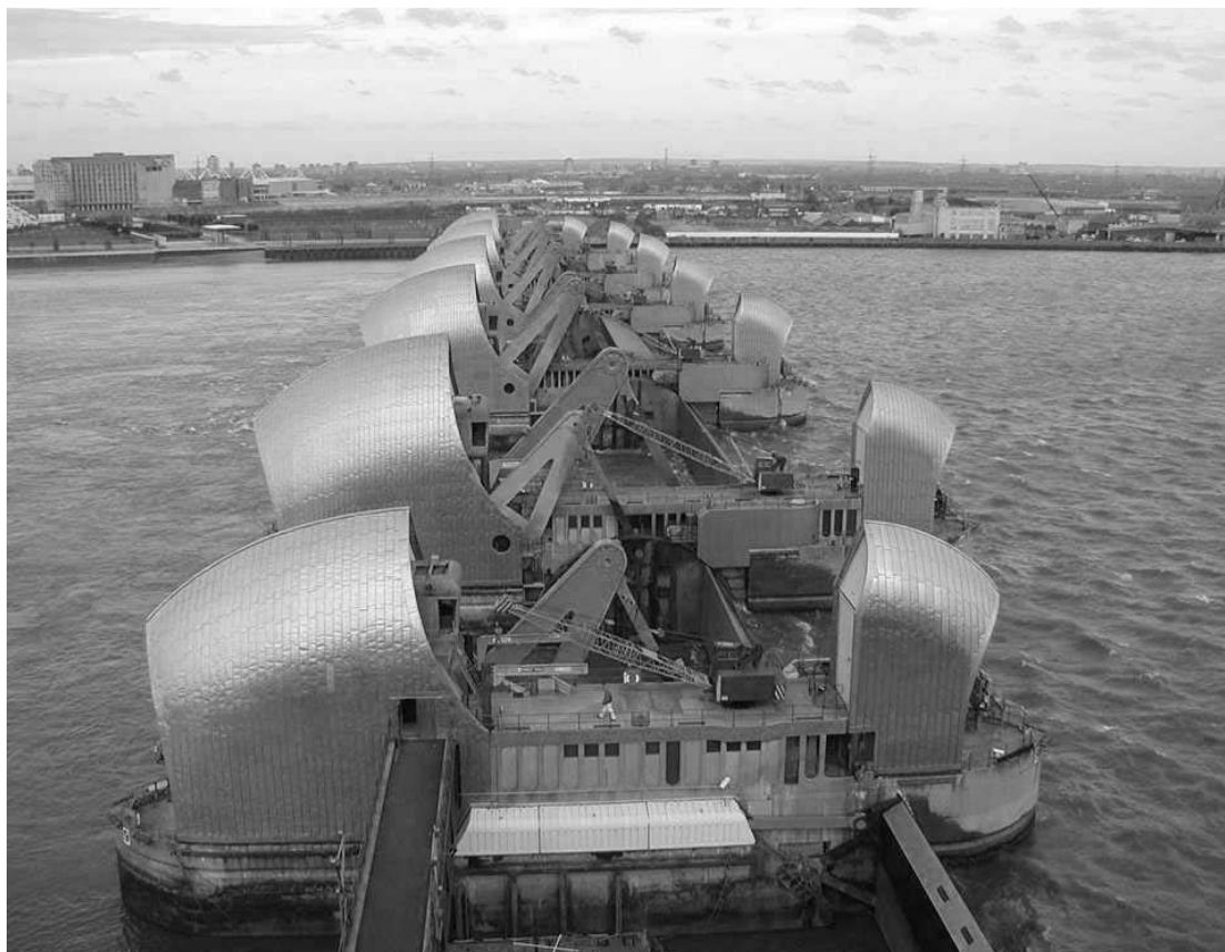
Figure 16. Thames Barrier, London (Photograph courtesy of the Environment Agency)
