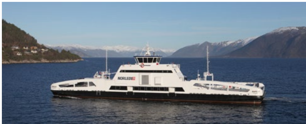
Since 2013, the MF Ampere , the world's first battery-propelled ferry, has provided a service across the Sognefjorden between Lavik and Oppedal. Photo: Norled
