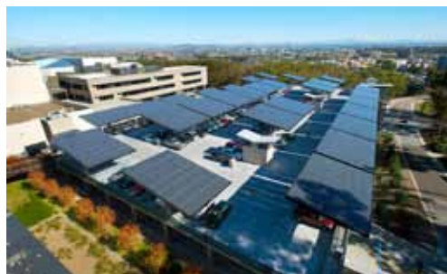
Solar panels such as the ones atop the Hopkins Parking Structure are part of the UC San Diego microgrid, which generates 92 percent of the electricity used on campus. Image: UC San Diego
