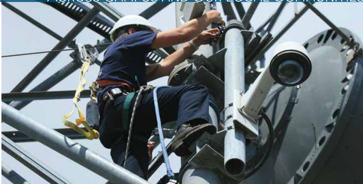
A Cal Fire firefighter installs an antenna on a microwave tower to connect a nearby fire station to HPWREN. Image courtesy of HPWREN/SDSC.
