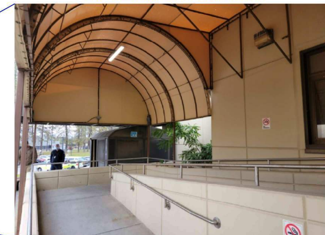
EXISTING SOUTH LIGHT AND ADA RAMP
