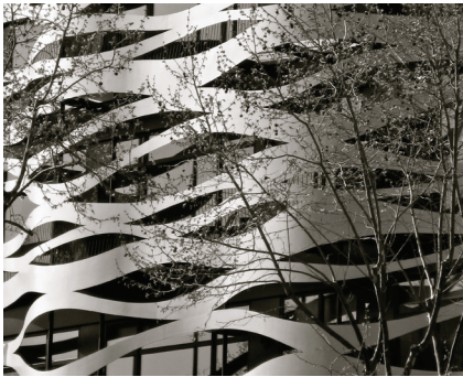
Facade renovation of Suites Avenue Aparthotel by Toyo Ito, Barcelona, Spain, is biomorphic in form, while enhancing the Dynamic & Diffuse light and shadows filtering to the interior space. Image © Aslaj/Flickr.
