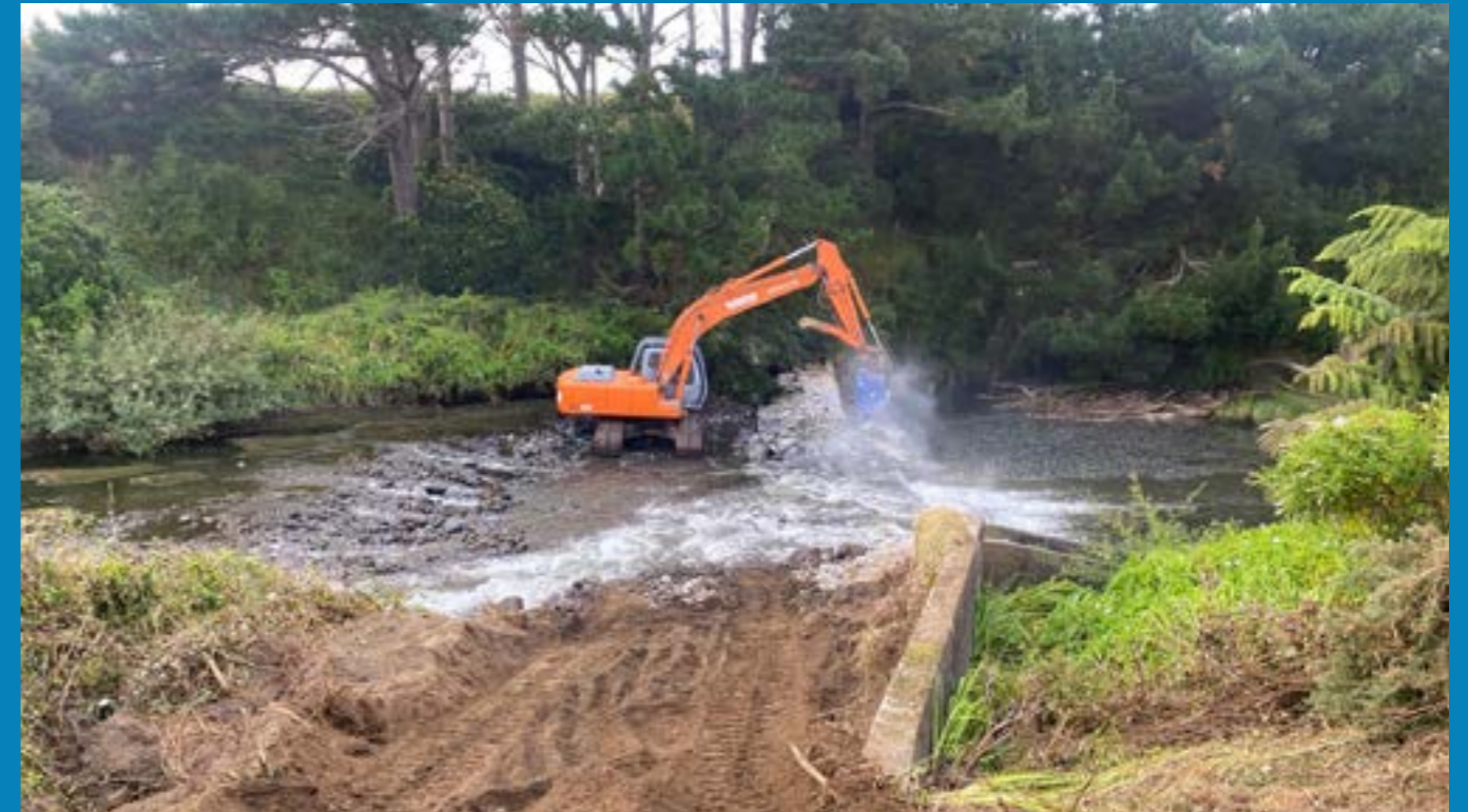
The removal of the weir was a huge milestone.
