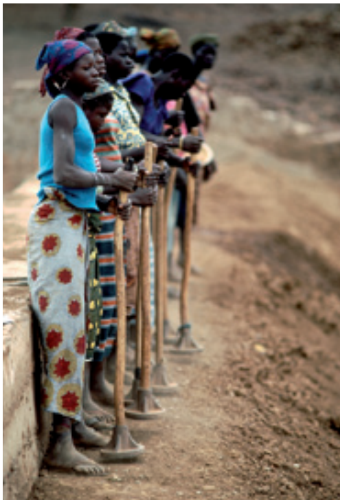
Women in Burkina Faso compacting the ground to stop the encroaching desert. UN Photo/John Isaac (flickr)
