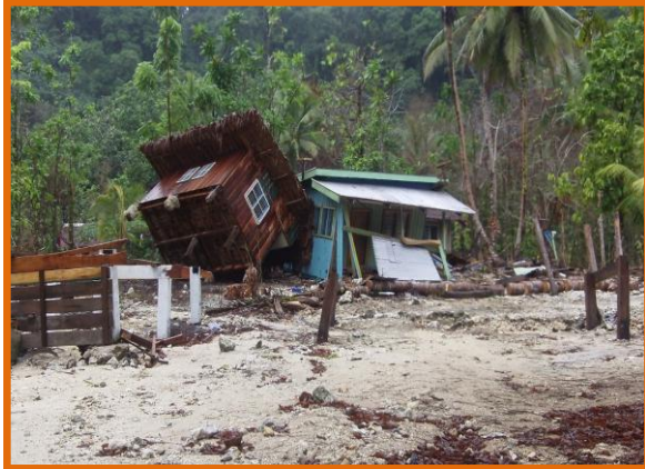
Damaged houses following tsunami on 6 February 2013, Temotu ©WVSI
